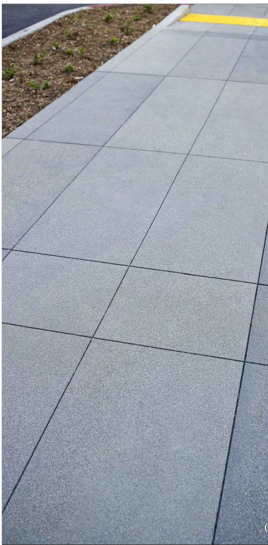
Sawcut concrete paving
